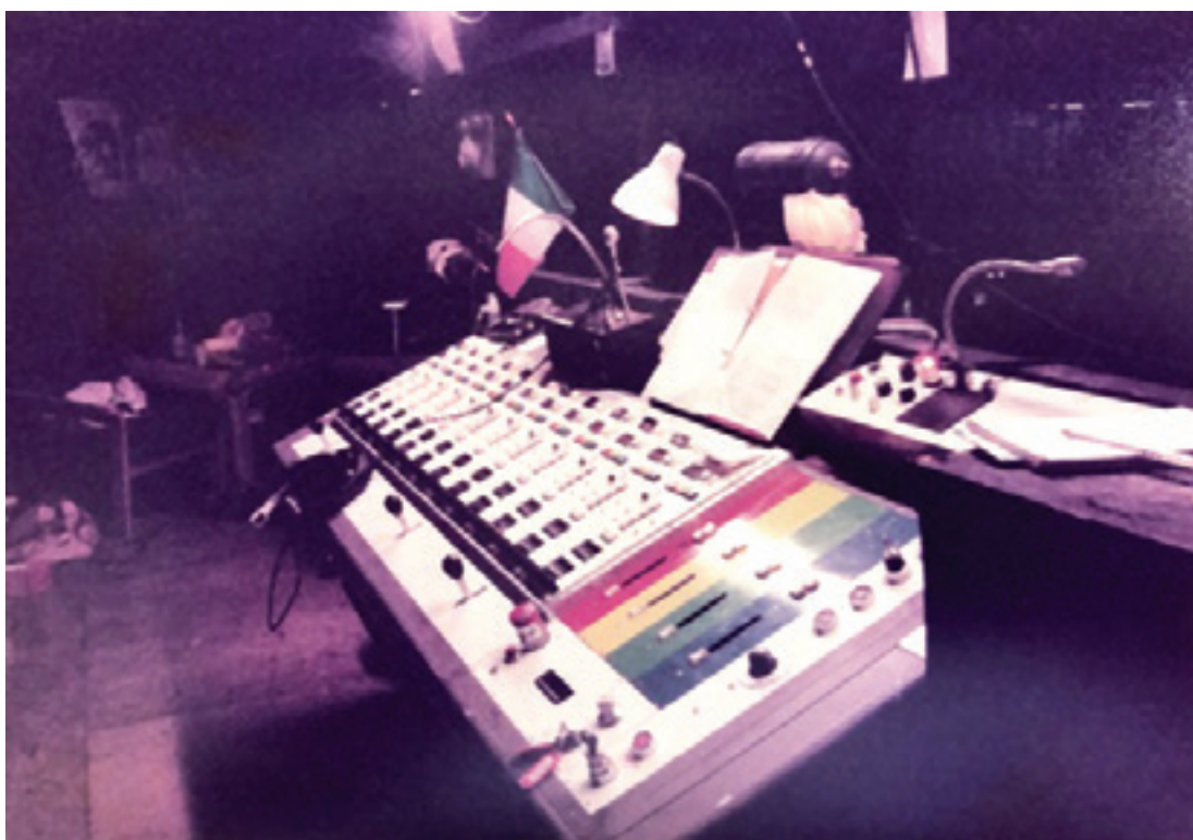
The automation control desk at the Barbican theatre 1983
